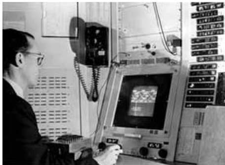
Ivan Sutherland at the console of the TX-2- Sketchpad Project, MIT, 1963 In 1963, his Ph.D. thesis, "Sketchpad: A Man-machine Graphical Communications System," used the lightpen to create engineering drawings directly on the CRT.
